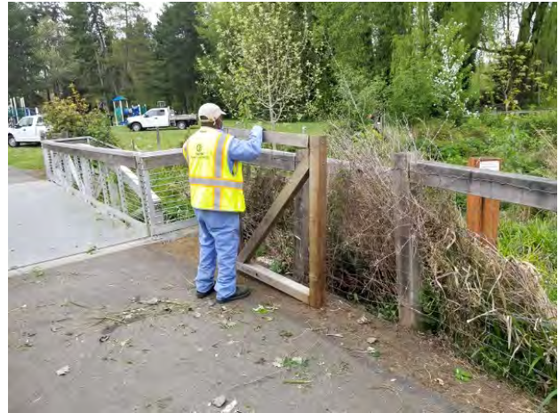
IMW repairing gate
